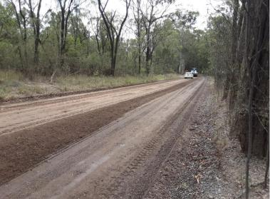
Photo 20 South-east facing view within the central portion of the study area depicting use of the road and undertaking unsealed road grading
