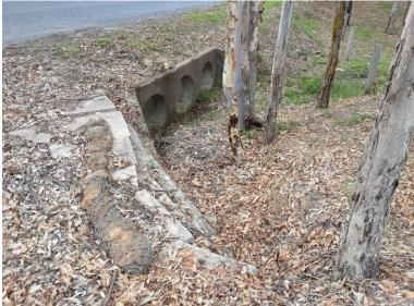
Photo 36 South-east facing view in the northern portion of the study area depicting triple pipe cement culvert
