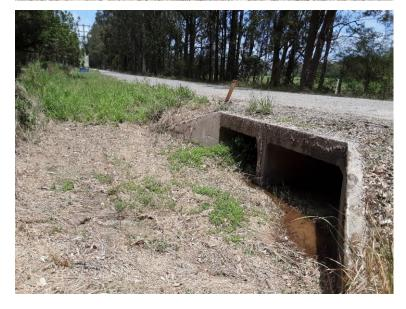
Photo 37 South-west facing view in the northern portion of the study area depicting double pipe square culvert
